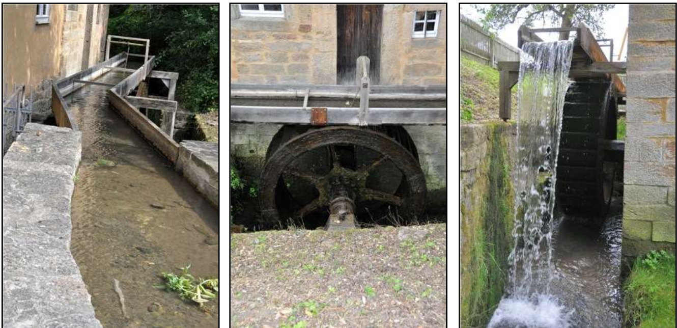
The Reß Mill: Left, the long water trough; center, the waterwheel with water flap; right, trough overflow
