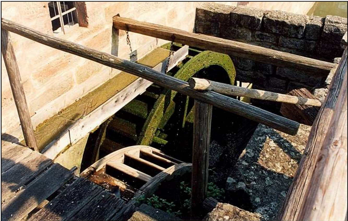
The water feed of the Unterschlaubach Mill in Northern Bavaria
